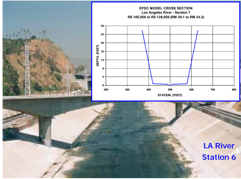
Figure 4: Photo and Cross-Section at LA River Station 6
