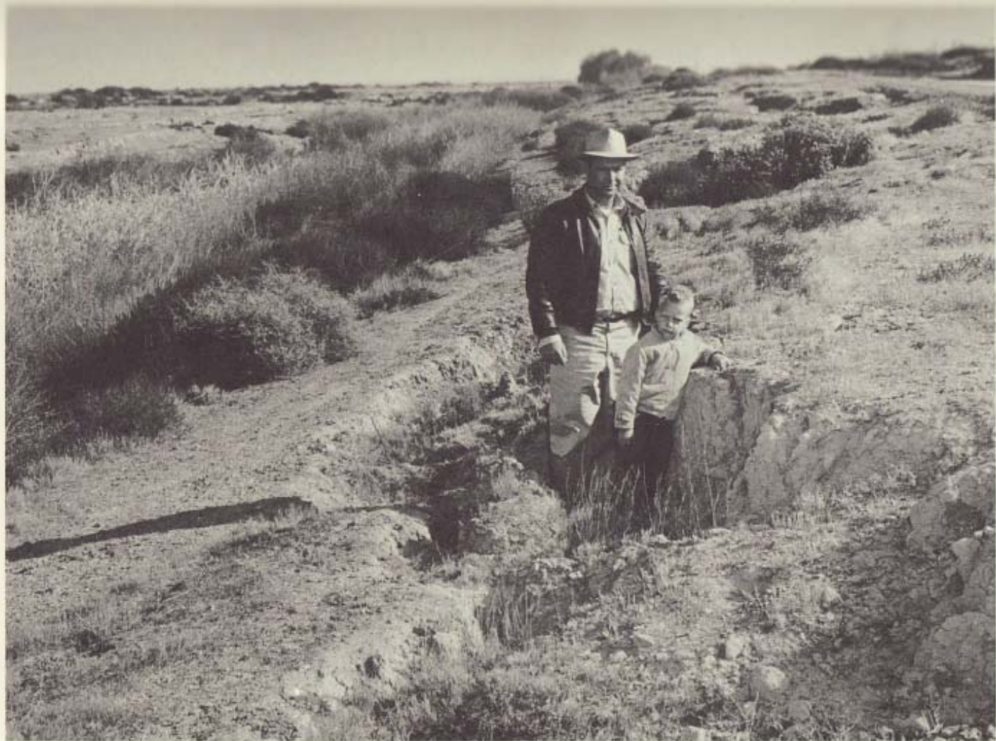
TYPICAL SUBSIDENCE ALONG ABANDONED IRRIGATION DITCH ( Photograph by California Department of Water Resources )
