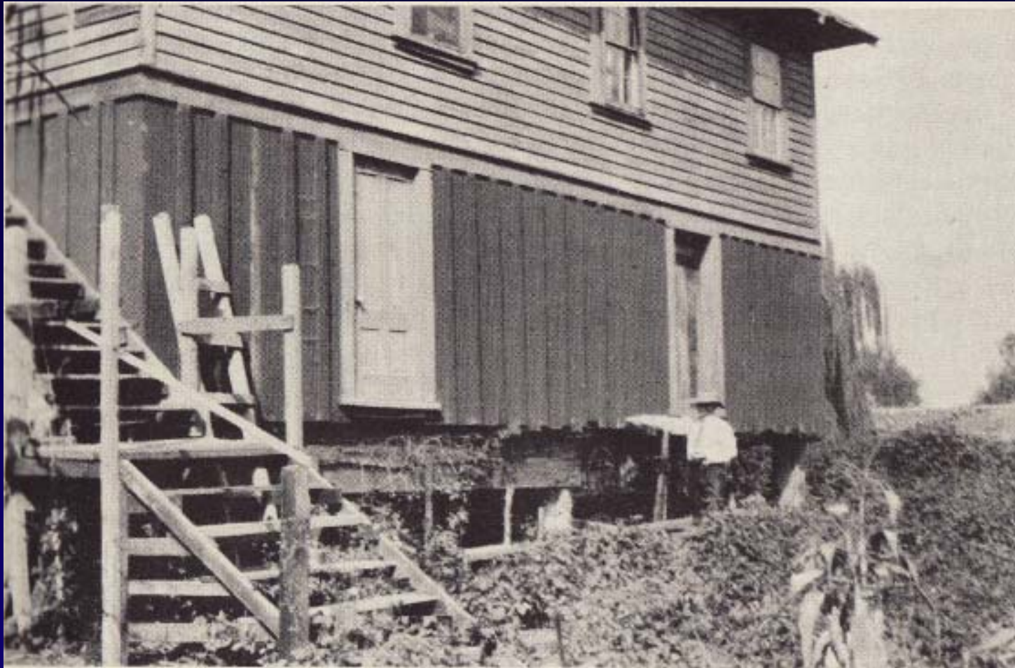
Fig. 10. The peat soil around this twenty-year-old house on Lower Jones Tract has subsided more than 4 feet. The pilings on which the house was built kept it from settling.
