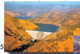
Pine Flat Dam
