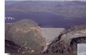
New Exchequer Dam
