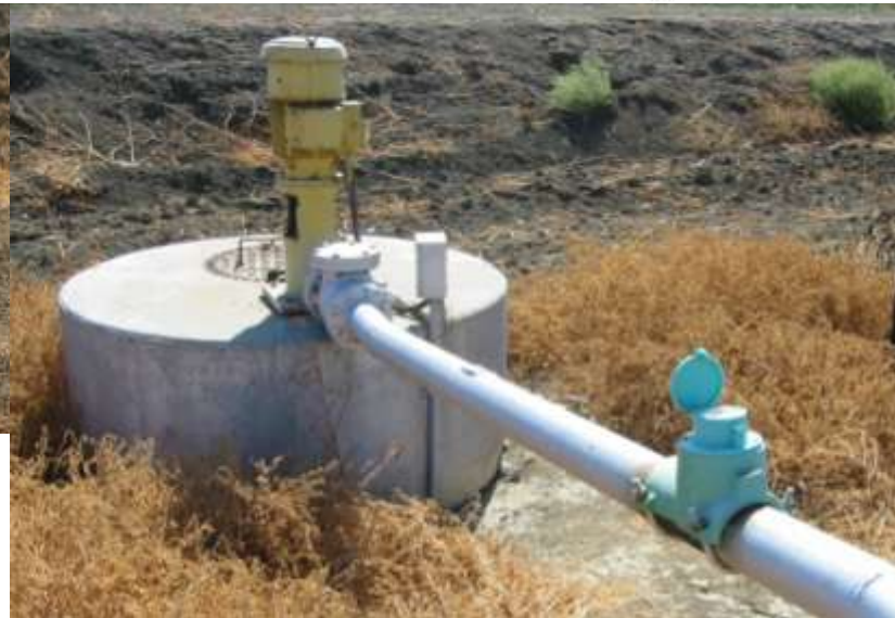
Drainage sump pumps in Panoche Water District Simulated water table depth monitor
